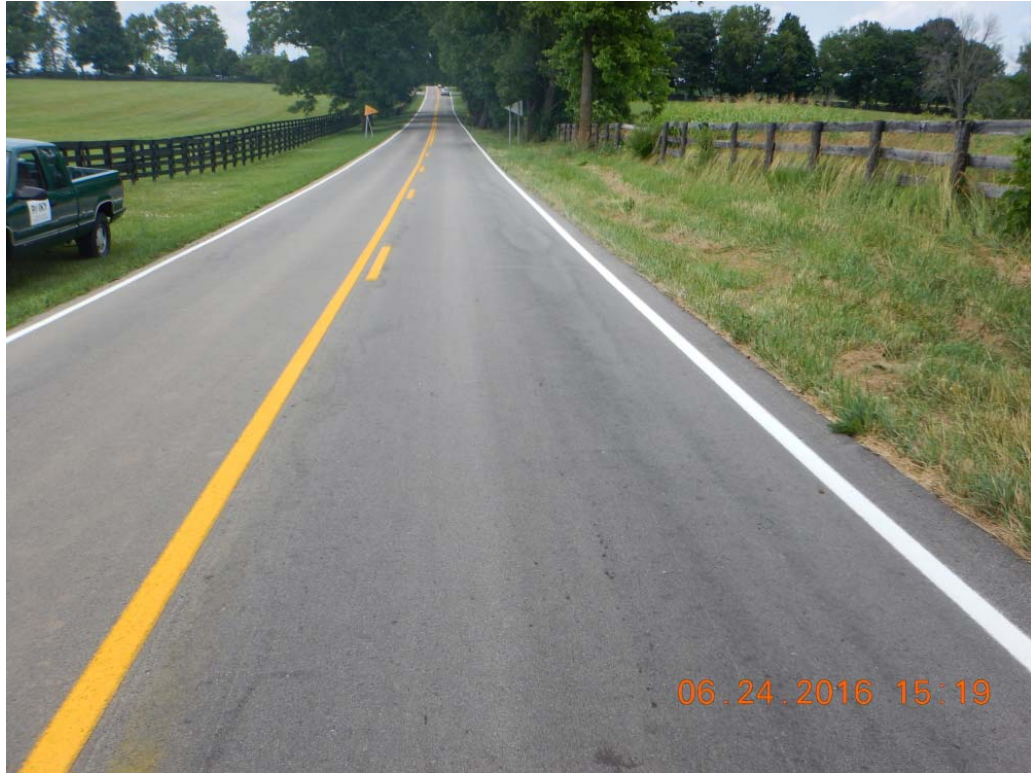
Figure 7.13: Fayette County, Surface Wearing, Microsurfacing
