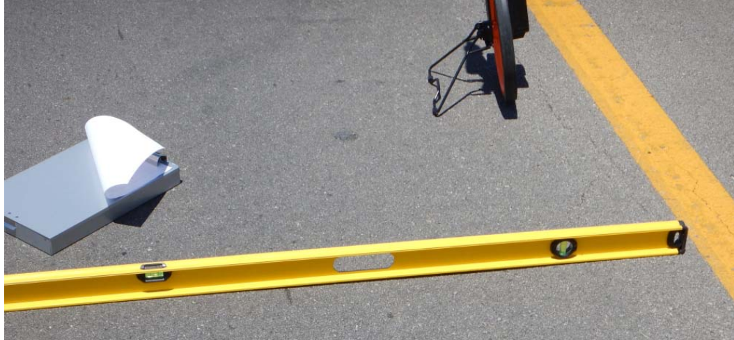
Figure 7.11: Nelson County, Rutting, Microsurfacing
